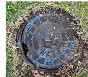
This is what your water main valve looks like. You can mark if you'd like but Jake will mark regardless.
